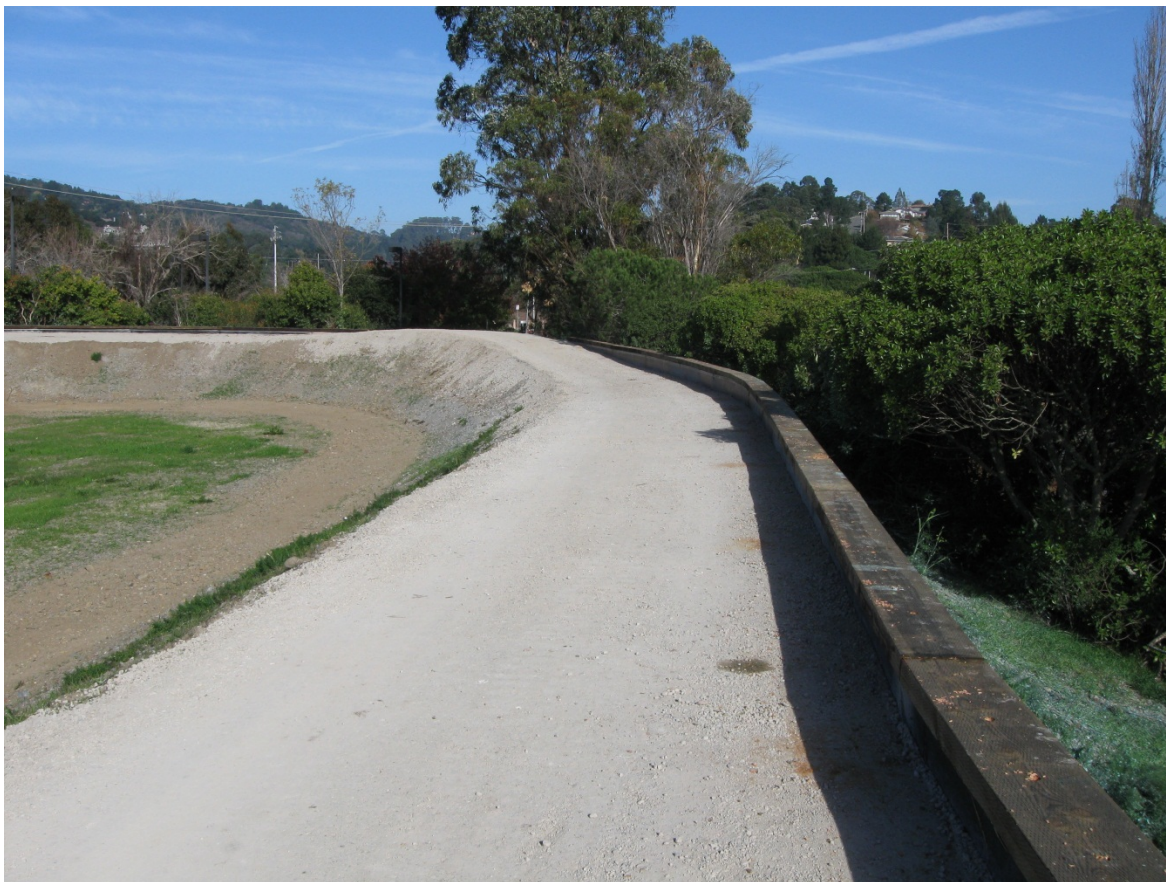
Figure 2: View of North Pond retaining wall and high berm for vehicular access to ponds.
