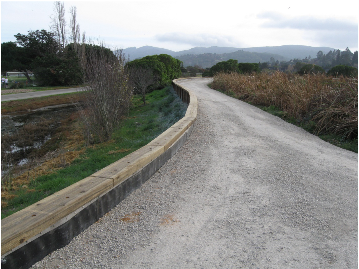
Figure 3: View of HDPE liner and wood wall next to the South Pond that provides wildlife viewing opportunities for local residents.
