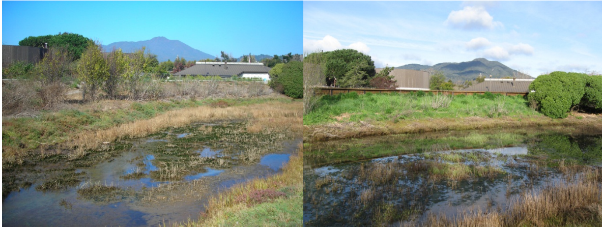
Figure 1: View of equalization pond berm before and after Nute Engineering Project in 2008 that more than doubled capacity of the ponds using a low-profile, HDPE-lined wood wall design. The tidal slough in the foreground was the location of sanitary sewer overflows in January 2008.
