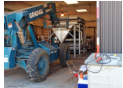
Installation of the Sludge Hopper
