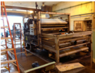
Demolition of the Existing Belt Filter Press
