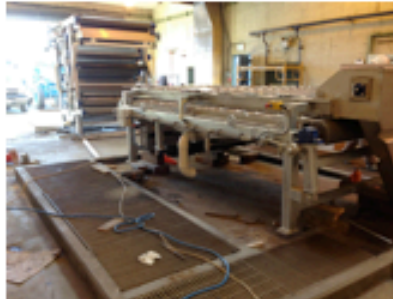
Installation of the New Gravity Table and Press Section
