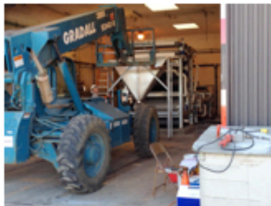
New Electrical Conduit and Washwater Piping
