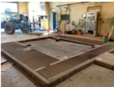
Complete Removal of the Existing Belt Filter Press
